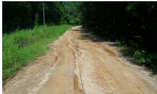
Our roads have become ditches exposing phone lines. The motor grader could have prevented these problems.
